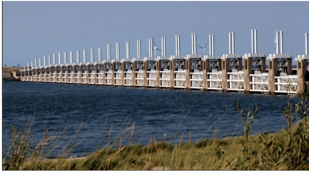
Figure 4.1.5 The modular design of the Eastern Scheldt Storm Surge Barrier 45 .
