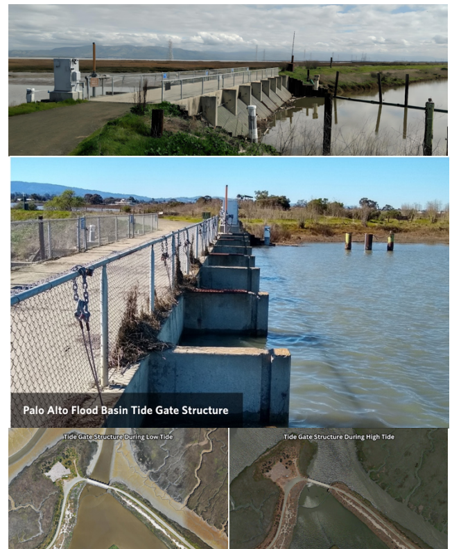
Figure 4.1.1 Images of PAFB's Tidal Gate Structure 39,40 . [Top]: The PAFB tidal gate structure from a ground-level view [Bottom]: The gate's operation during low tide (left) and high tide (right).
