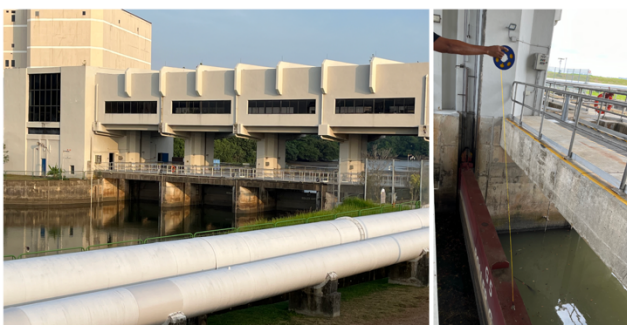
Figure 2.1.4 [Left] Close-up of the Older Pandan Tidal Gates (Reservoir-Facing) [Right] Height measurement of the newer tidal gate that were built higher for current tide levels.
